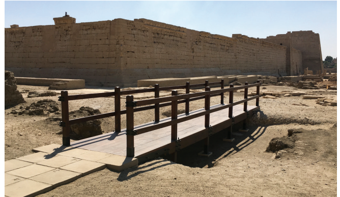
Completed bridge, April 11, 2019. Photo: Ray Johnson.
