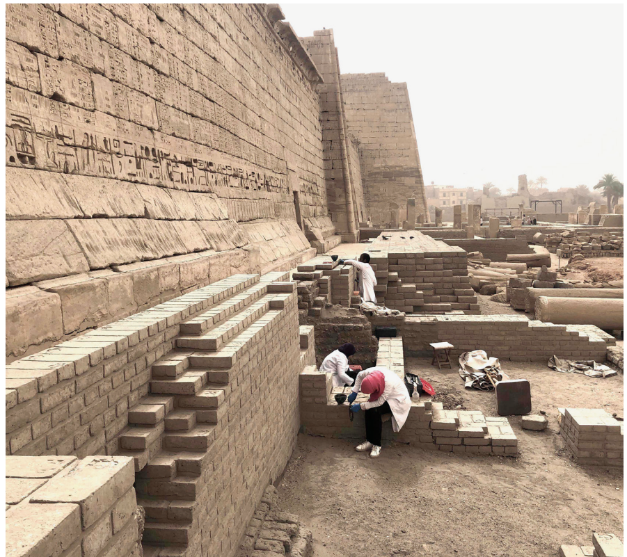
Conservation team working on mudbrick restoration, March 2019. Photo: Lotfi Hassan.
