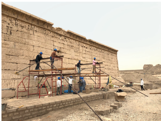
Pavement and brick work on the northern side of the Ramesses III mortuary temple, March 2019. Photo: Frank Helmholz.
