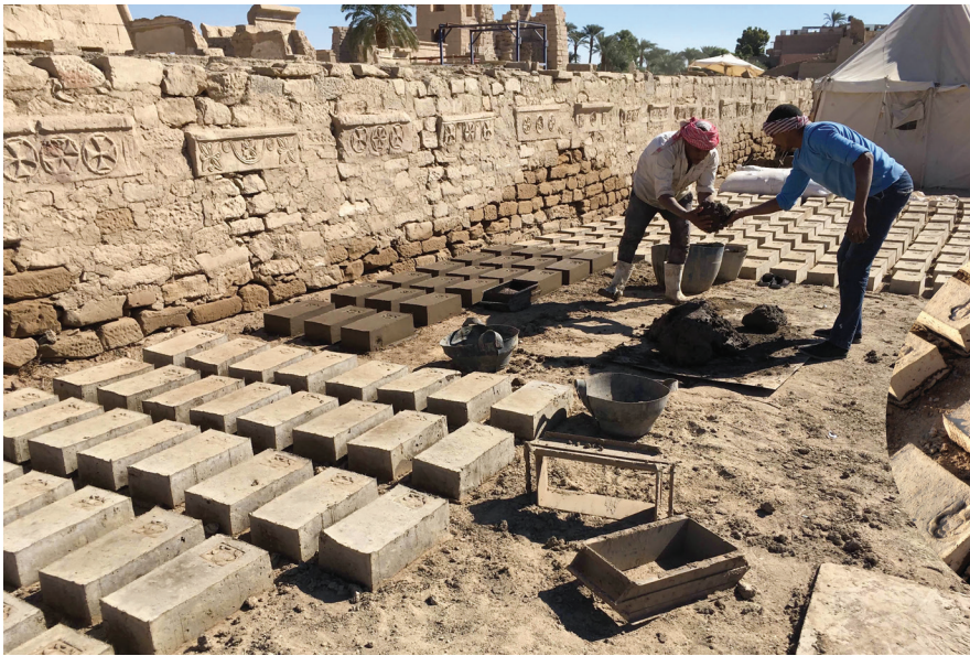
Restoration brickmaking, Medinet Habu, December 10, 2018. Photo: Ray Johnson.
