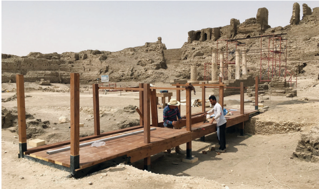
Bridge nearing completion, March 23, 2019. Photo: Ray Johnson.
