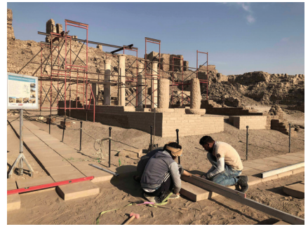
Butehamun House pavement installation, January 2019. Photo: Lotfi Hassan.
