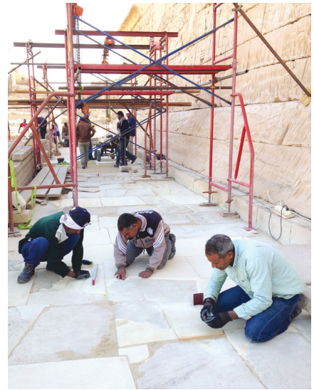
Slab edge smoothing, December 29, 2018. Photo: Ray Johnson.
