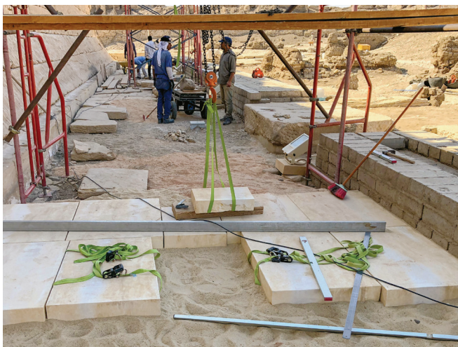
Pavement laying in the western sector, April 1, 2018. Photo: Frank Helmholz.
