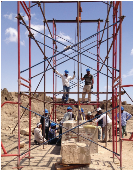
Western High Gate block group being assembled, March 25, 2019. Photo: Ray Johnson.
