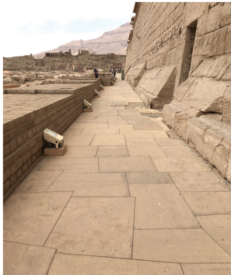
Finished pavement restoration, southern side, February 13, 2019. Photo: Ray Johnson.
