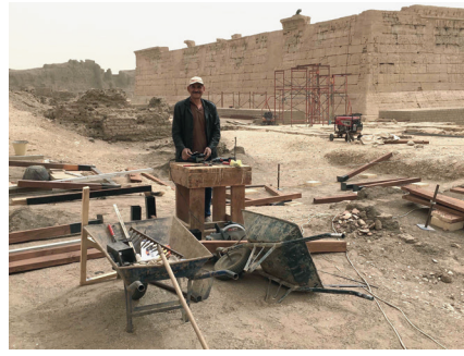
Chicago House carpenter Samy preparing bridge parts, March 14, 2019. Photo: Ray Johnson.
