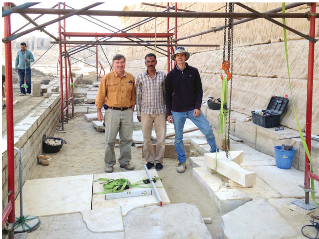
Frank, Saber, and Johannes laying stone slabs, February 27, 2018. Photo: Ray Johnson.
